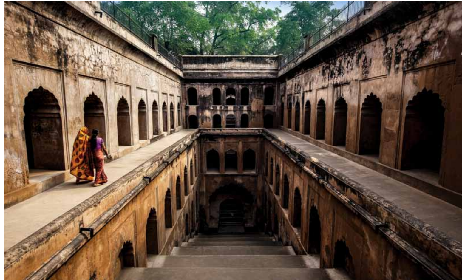
(Clockwise from above) Kali Bari is one of the oldest temples in Lucknow; washed clothes hang to dry along the Gouti River; the Radha Krishna Temple; the bowl of Bara Imambara, built in a pure Indian style, was once used as a water reservoir.
